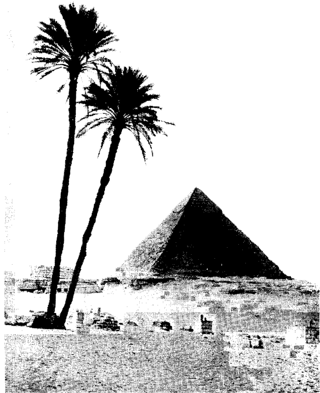
The pyramid of king Khafre (Kha-f-Ra). This is the second-largest of the three great pyramids of Giza, which were built during the IVth dynasty, between 2686 and 2613 B.C. It has a perpendicular height of 447-1/2 feet. At the top a fragment remains of the original coating of limestone and unpolished granite slabs.
